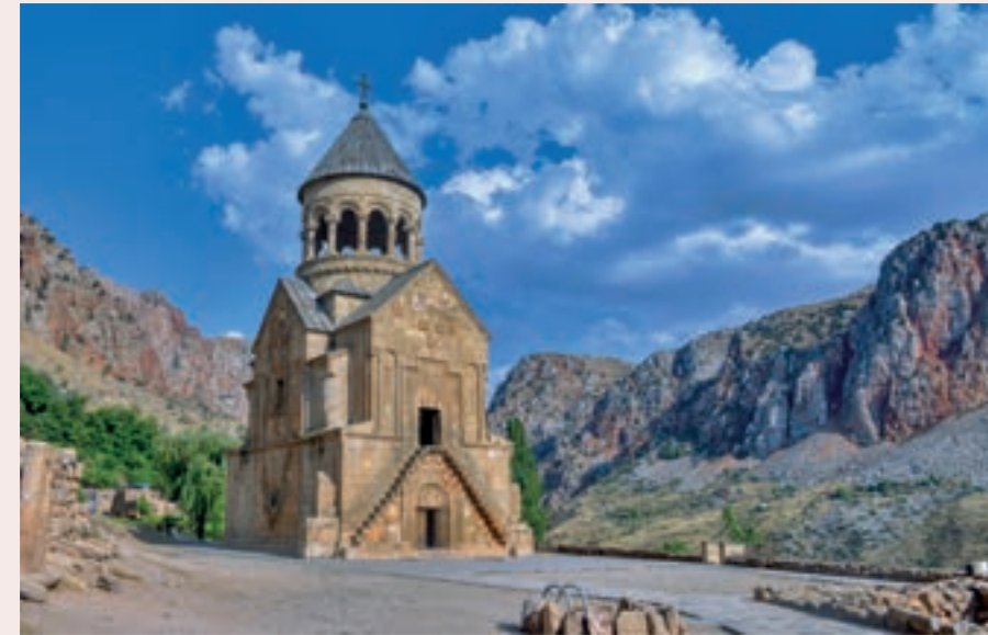
Fig. 13. St. Astvatsatsin church from the west (photo: Tigran Apikyan, 2021)
