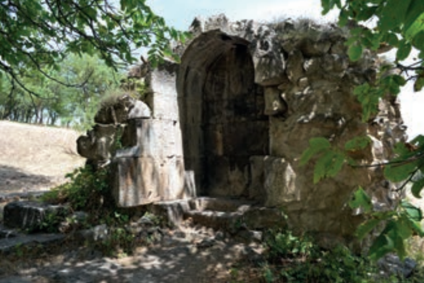
Fig. 2, The partially dilapidated memorial sanctuary from the southwest (photo: A. Harutyunyan, 2021)
