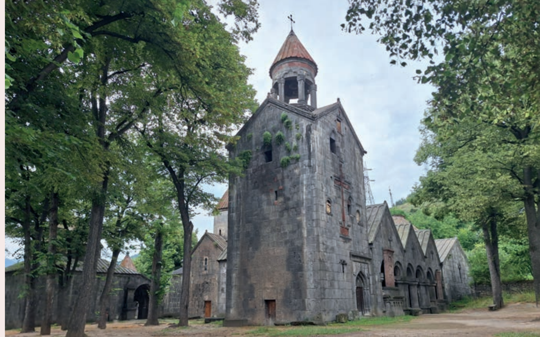
Fig. 1. The courtyard of Sanahin monastery (photo: Khachik Harutyunyan)
