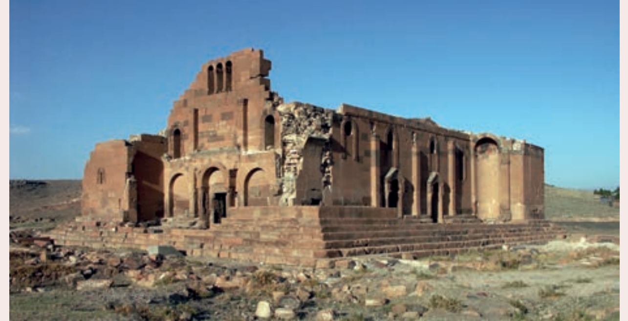
Fig. 2. Yereruyk, basilica. General view from the southwest (LA3M, 2012), (photo: Patrick Donabédian).
